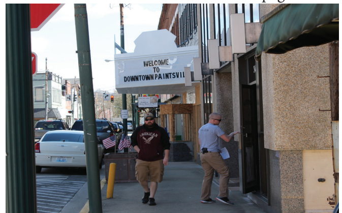
Downtown Paintsville’s historic Sipp Theater is getting a facelift, and going back to its original look. The box office is being reconstructed, and a close model of the original marquee hangs over the sidewalk again.
